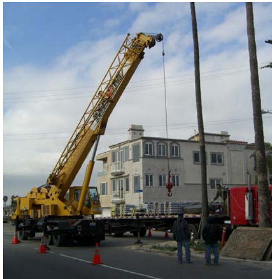
Crane Moves into Place to Erect the Rock
